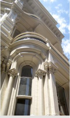
The original slate shingles on the mansard roof were reinstalled wherever possible. The finials (left) were restored, or replaced where missing with fiberglass replicas, and a large structural crack in the pavilion was repaired (center). Decorative cast iron facade elements, such as column and pilaster capitals (right), were also restored to their original beauty.
