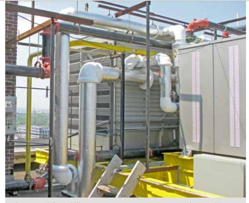
After ground-floor chillers at 135 Montgomery Street were destroyed by Hurricane Irene in 2011 and then Superstorm Sandy a year later, new replacement chillers were relocated on the roof and placed on a reinforced steel platform.
