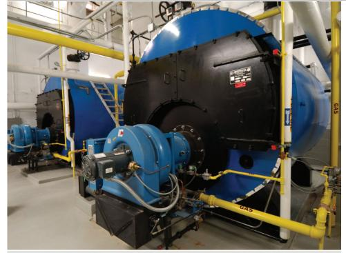
The board at 75 Henry Street replaced the building's original steam boilers, which were nearly 40 years old, with these new Scotch-marine steel boilers.
