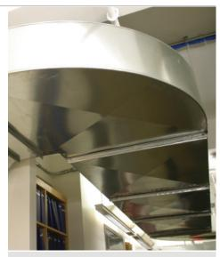
The suspended ductwork system, including supply and return air trunks and branches, provides effective ventilation throughout the office.
