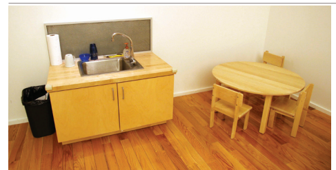
Classroom sinks have self-contained ejector pumps for better drainage.
